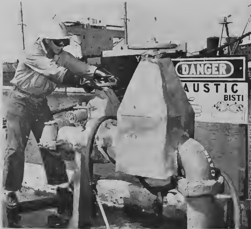
BEFORE opening a caustic valve the employee dons goggles, gloves, stands on a wooden board and uses wash water.
